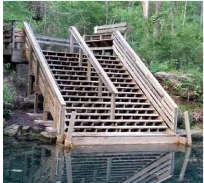
Steps rebuilt; Handitreads added and an additional ladder installed.
